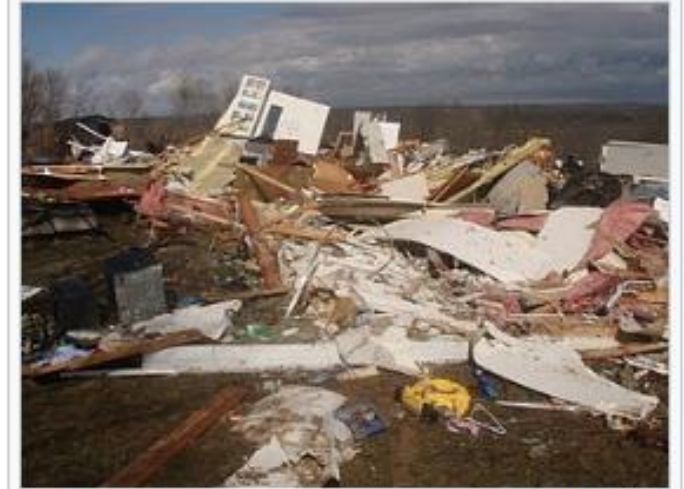
This mobile home was destroyed by a relatively weak EF0 tornado.
